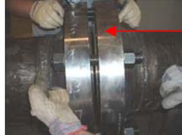
8. Apply dry film lubrication to 50% of the nuts only and allow to dry for 1 hour. Mark front of nuts with white paint stick. (See Appendix A)
